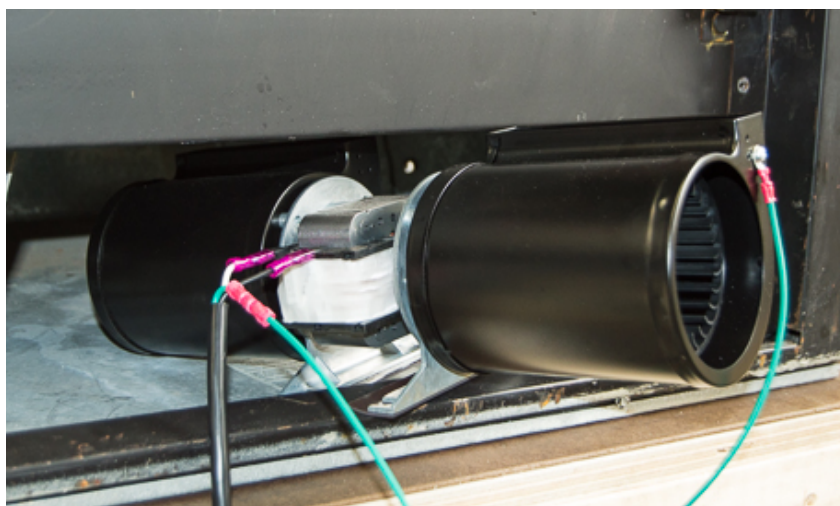
Figure: 1 • Does not matter which metal tab you connect the black and white wires to.
